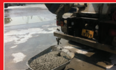
3. Concrete mixed in
