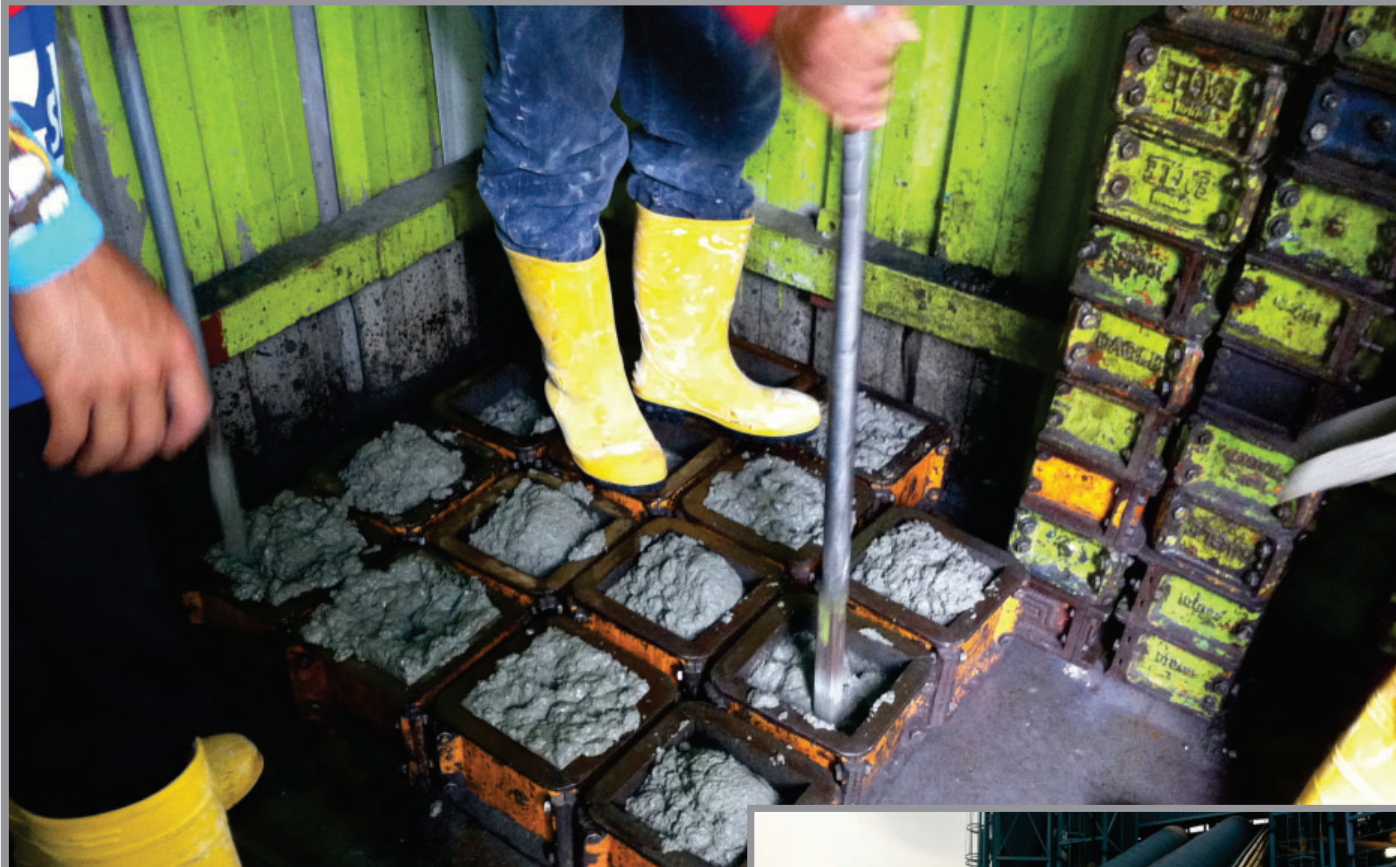
◀ COMPACTING CONCRETE CUBE
