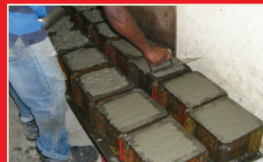
6. Preparation of concrete cube
